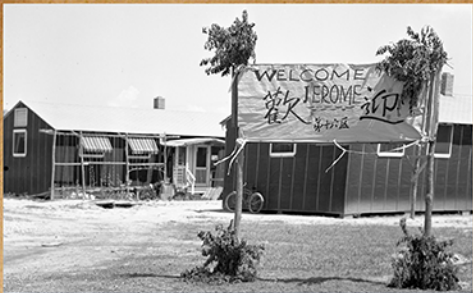
Jerome, Arkansas, housed many of the Fresno County internees from September, 1942 through mid-1944. Uprooted once again, prisoners were forced to relocate to Rohwer. Here, a sign erected by earlier residents of Rohwer welcomes the new arrivals from Jerome - June 21, 1944. Charles E. Mace, War Relocation Authority
